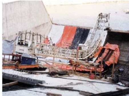
(b) St. Mary's Dam, Alberta
