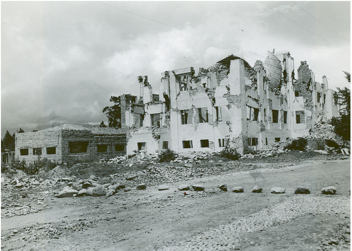
Figure 1.1: Collapse of a building under earthquake [1]
